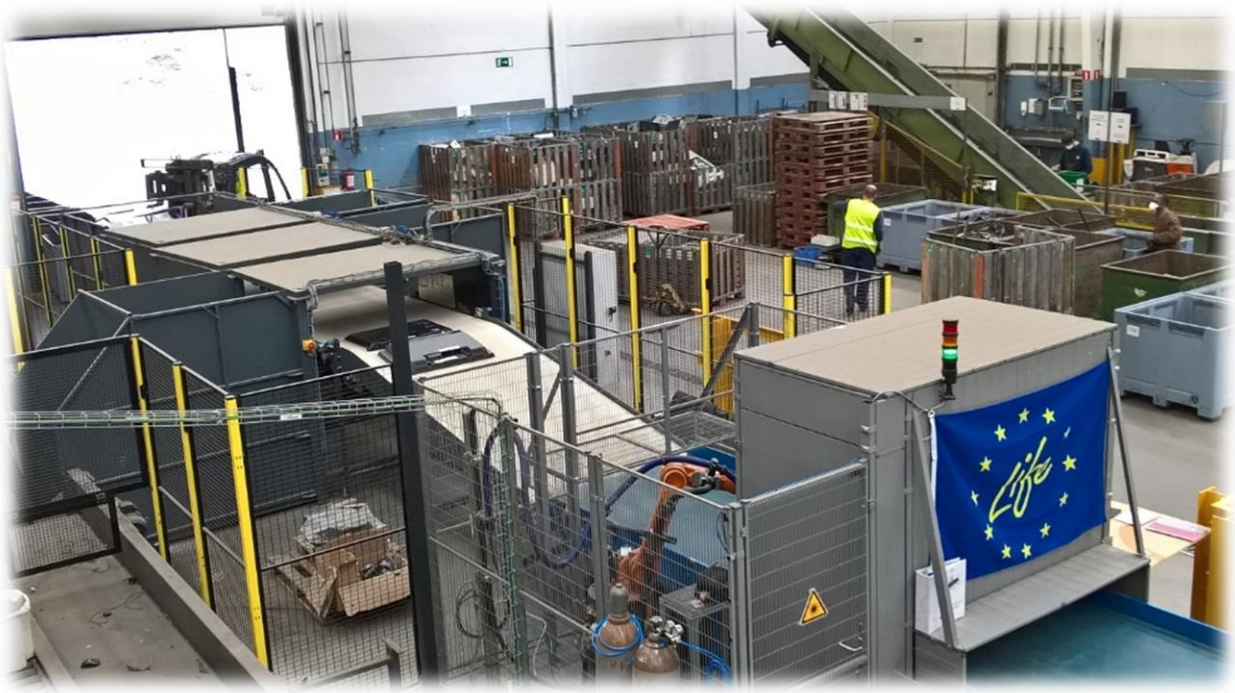
Quantum InLine installed in the recycler site, July 2018
