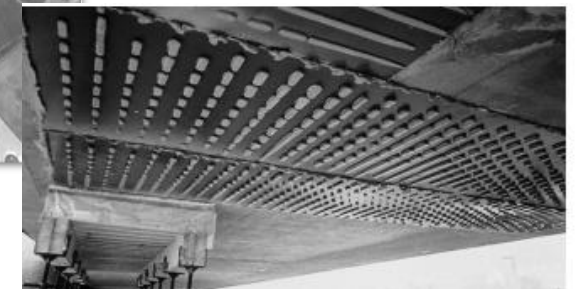
Renforcement composite Renforts collés acier ...
